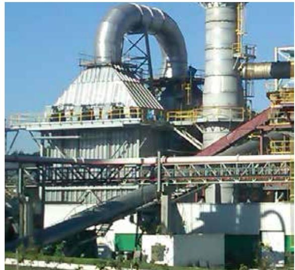
*Particleboard dryer wet ESP system*
