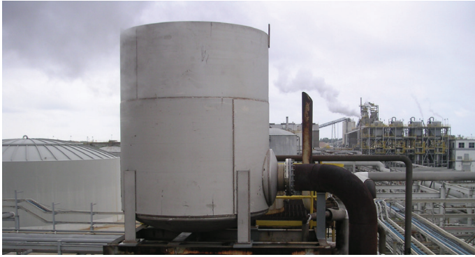
» Vent silencer at a Midwest phosphorus plant
