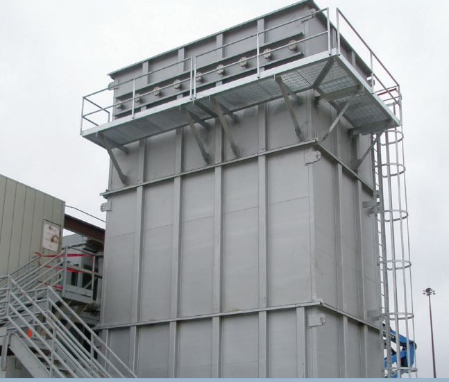
» Dür Universal designed and manufactured this exhaust system for a Westinghouse 251 gas turbine
