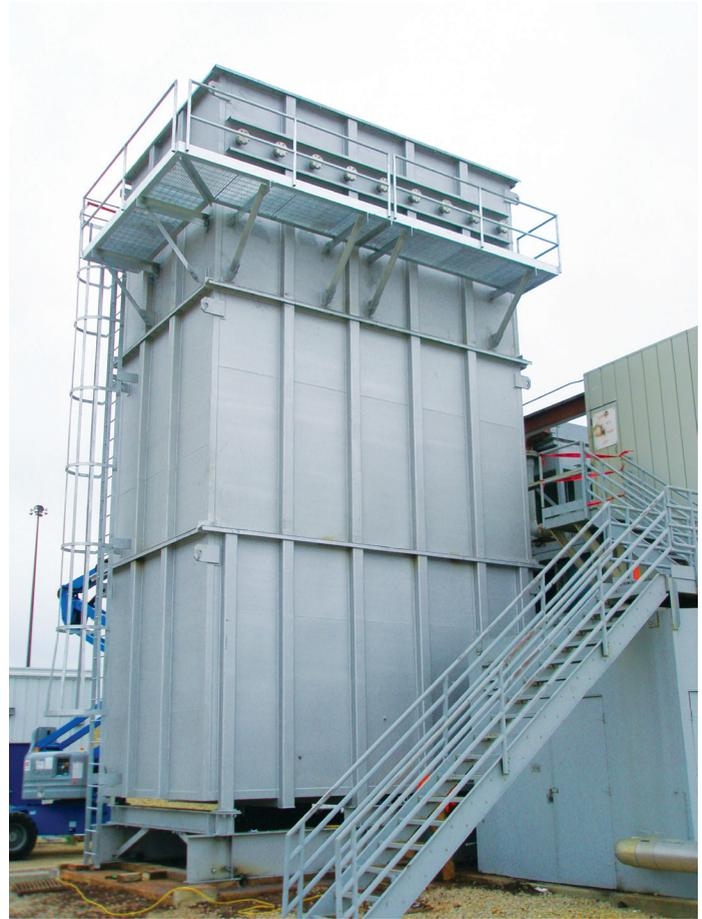
Dürr Universal designed and manufactured this exhaust system for a Westinghouse 251 gas turbine power generation peaker unit. The original unit experienced significant deterioration to the inside liner sheets and exhaust baffles.
