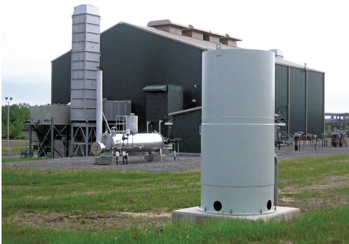
Turbine exhaust silencer and vent blow-down silencer at a gas compression station
