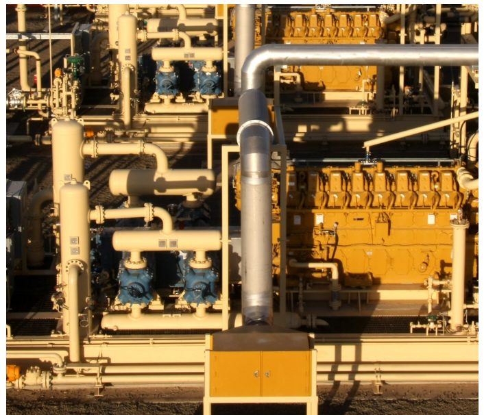
Gas gathering and compression: reciprocating engine exhaust silencers and emission solutions
